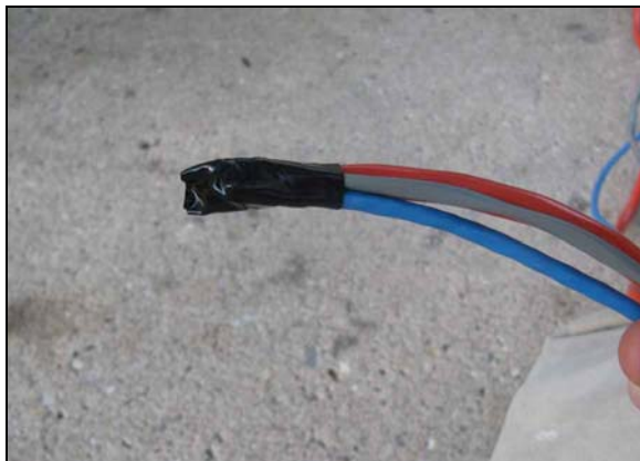
Figure 21: Tape Three Cable Ends
