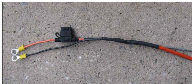
Figure 17: Completed Power Connection
