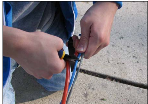
Figure 20: Cut Three Cables to the Same Length
